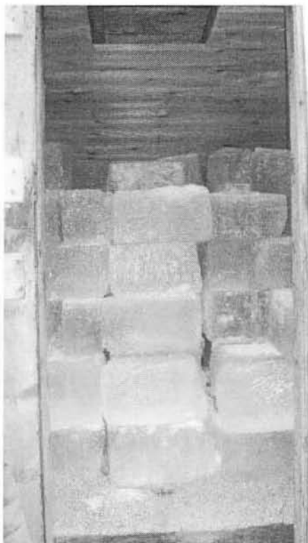
Ice packed into the ice house February 2, 2008. We added a few more layers of ice and then packed sawdust around the edges and on top after this picture was taken.
