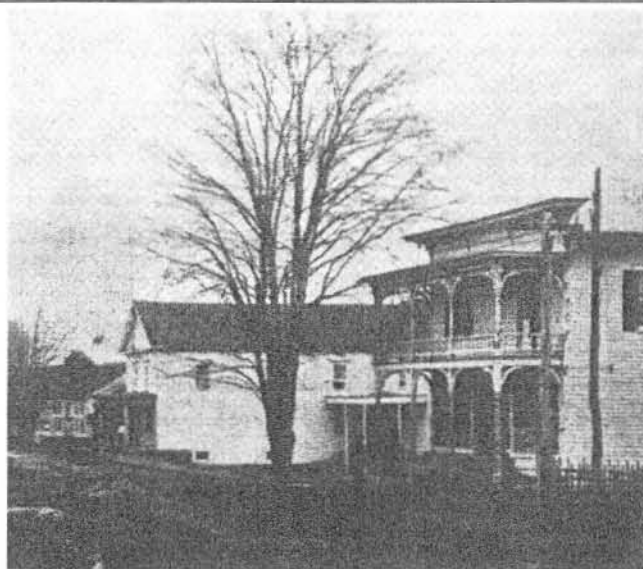
This photograph, c.1900, shows the former Levi Hanford store (left) in its new position in the center of the village and the Henderson store (right) built in 1890. It was comparatively easy to move post and beam style buildings like the old Hanford store.
