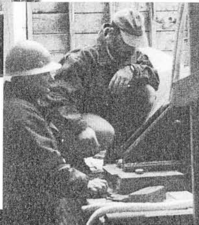
→ 4. The boiler sits on 4 "feet" that slide on graphite pads. As the boiler heats and cools, it will expand and contract on these pads, so we had to get it set right.
